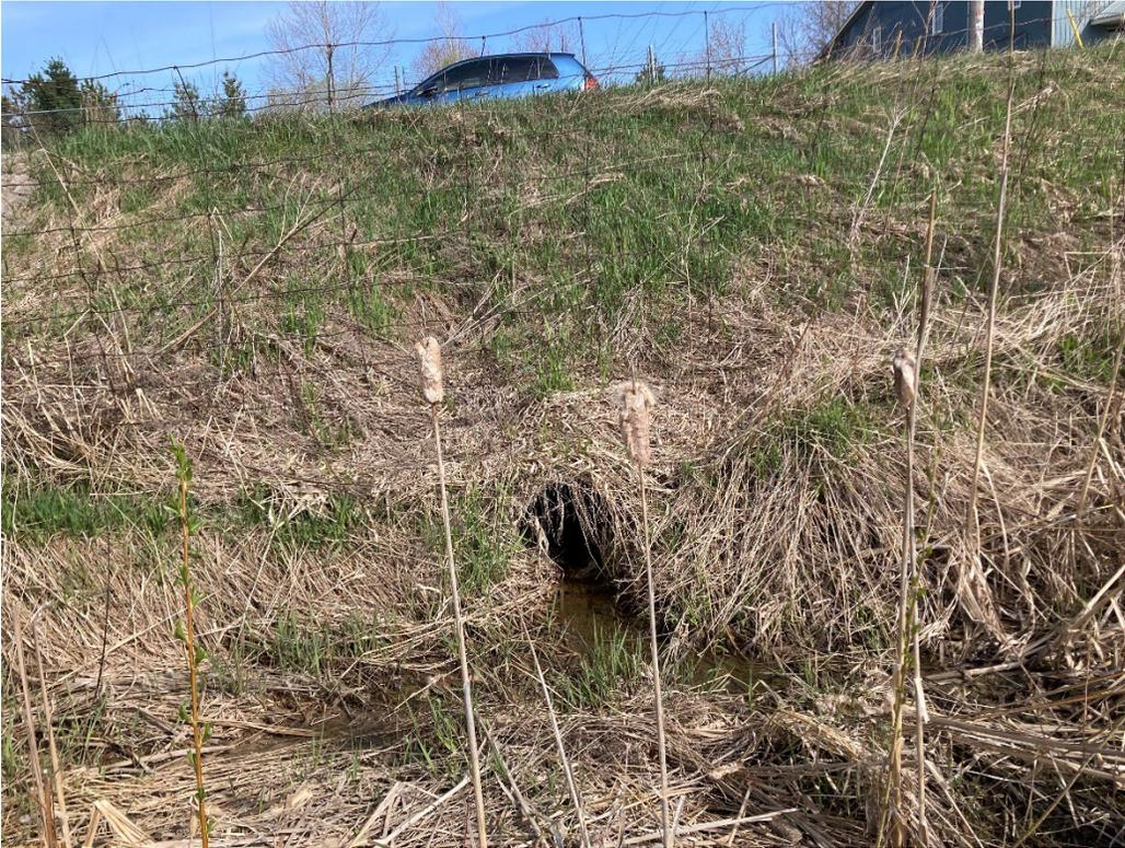
*Image 1 Existing Culvert Northwest 450mm Inlet*
