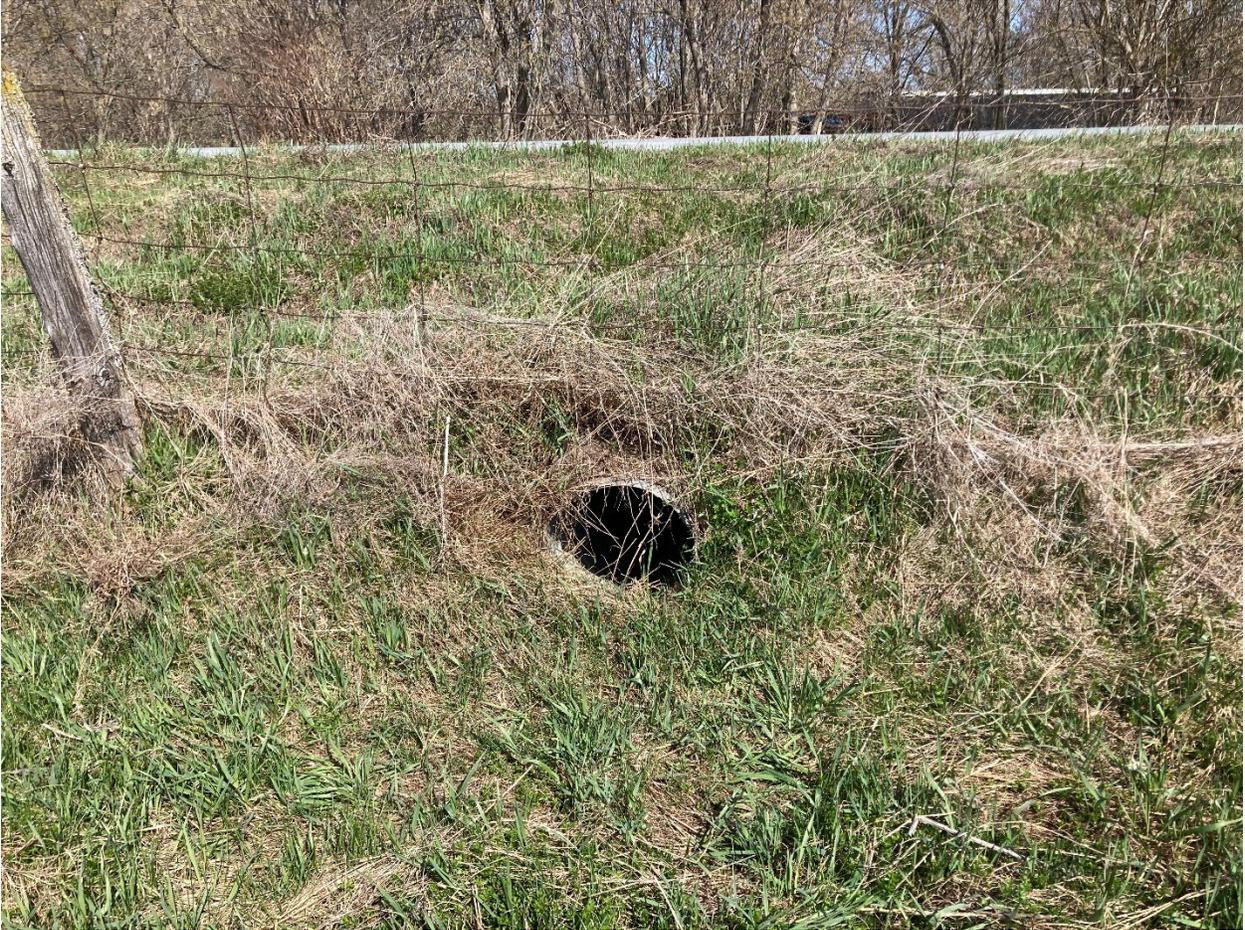
*Image3 Existing Culvert Northeast 400mm inlet*
