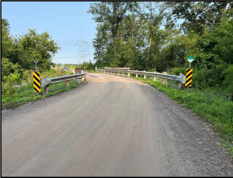
Roadway looking west
