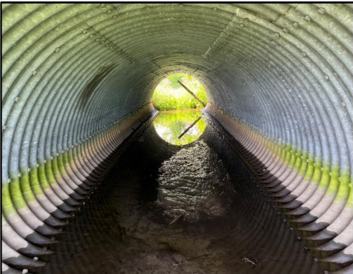
Looking south through barrel
