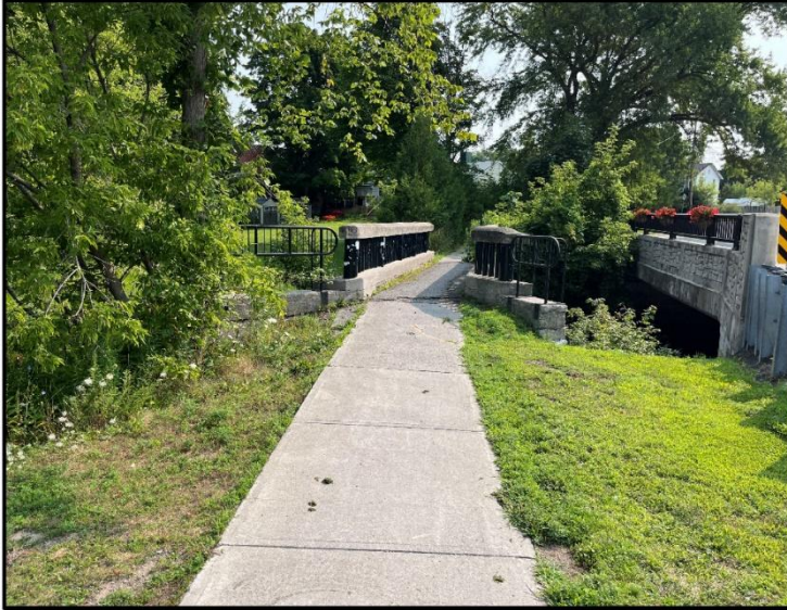
Walkway looking east
