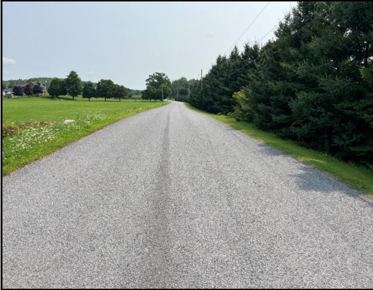
Roadway looking east
